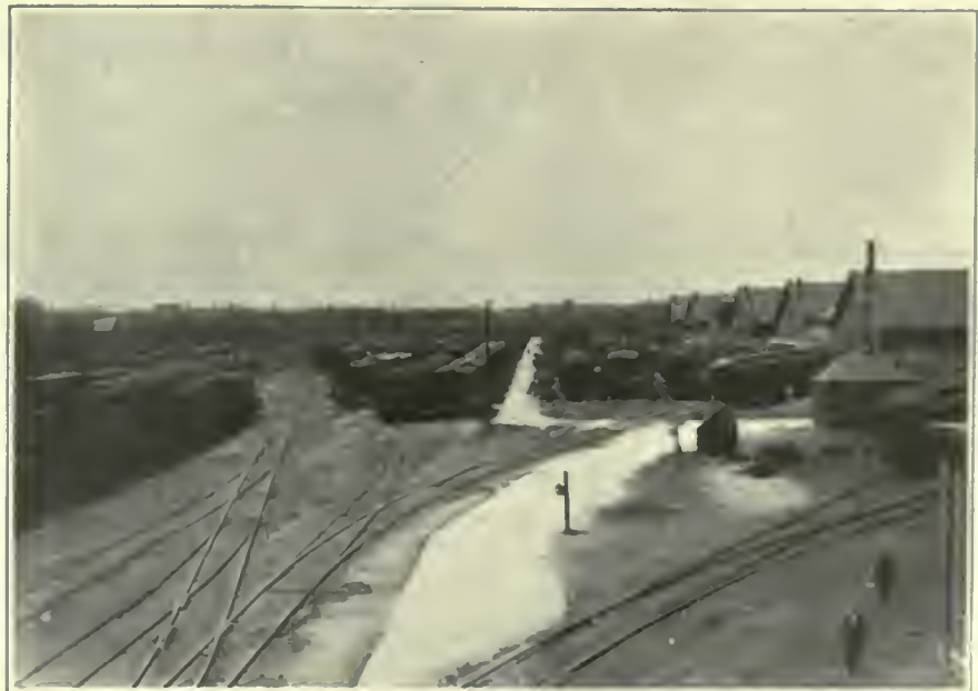
FIG. 343. MISCELLANEOUS YARDS. General View of Freight Car Repair Yard of the Chicago & North Western Railway at the 40th Avenue Yard.
